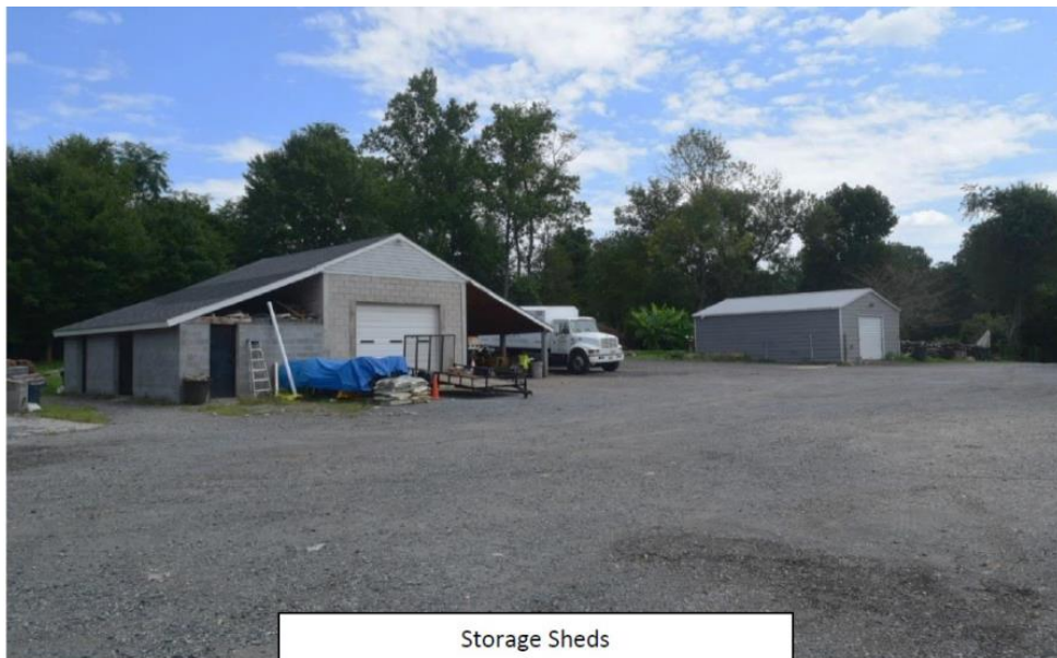
Figure 10: Existing Storage Buildings
