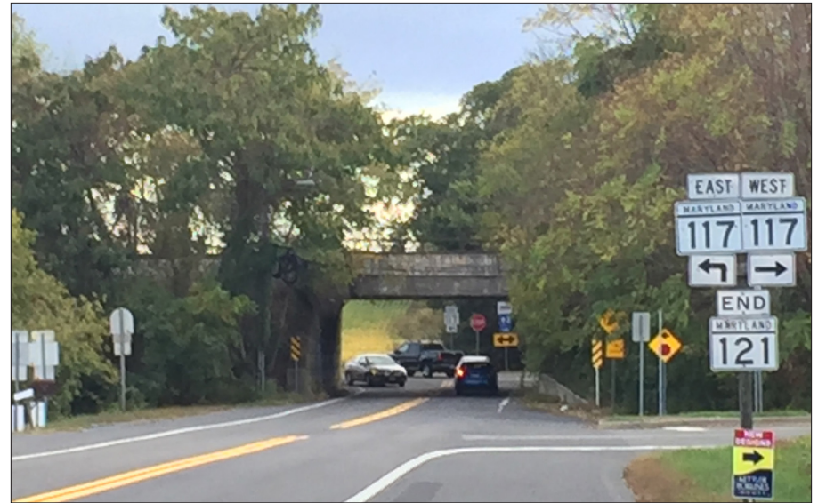
Existing underpass beneath railroad tracks in Boyds
