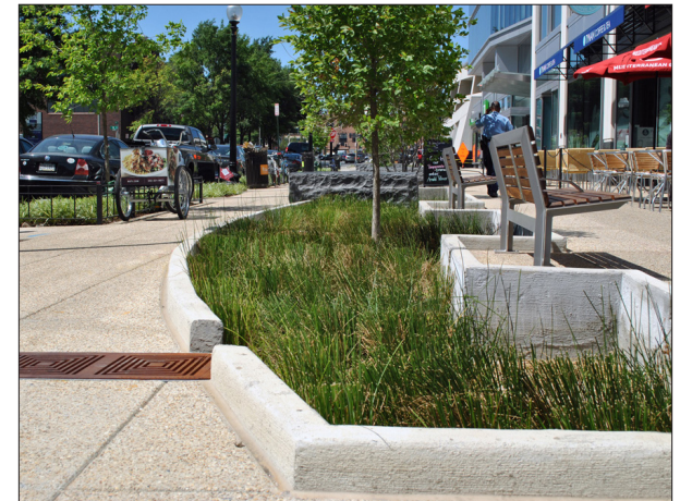
Planted area on sidewalk for stormwater management
