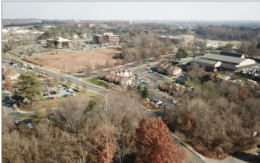
Germantown MARC Station area north of the railroad tracks along Walter Johnson Road
