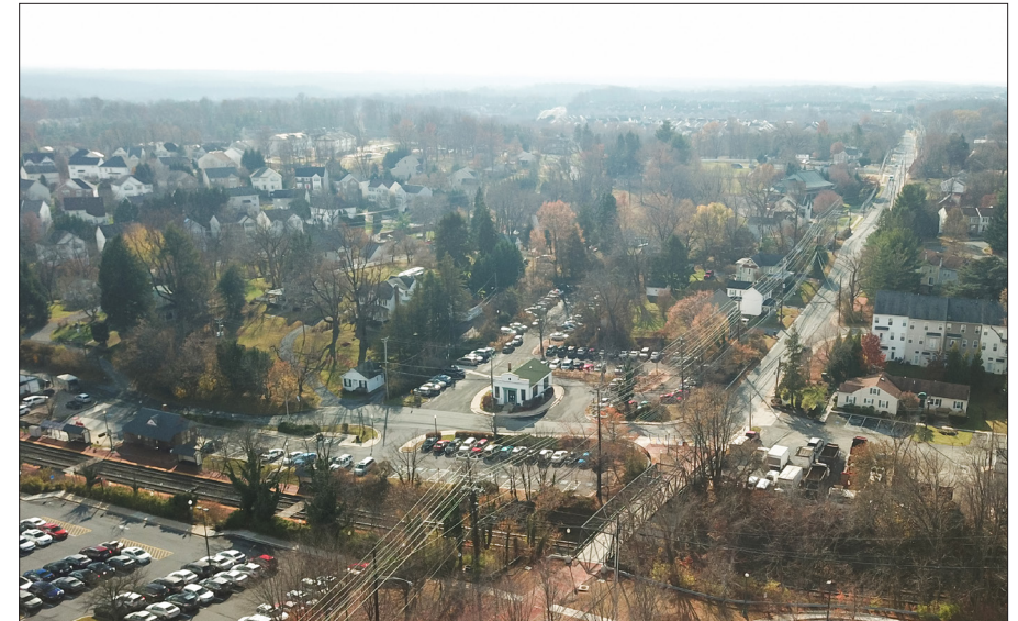
Germantown Historic District and residential area south of the railroad tracks
