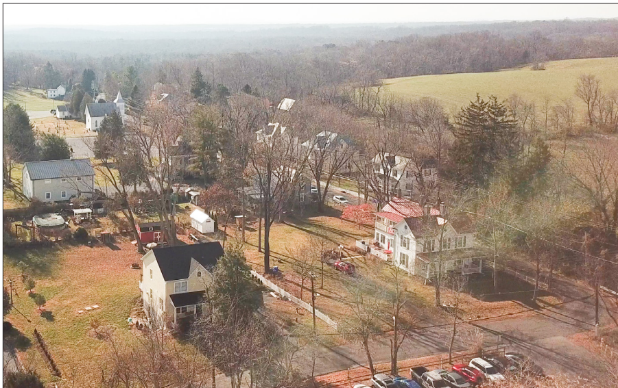
Historic houses and Boyds Presbyterian Church (upper right corner) along White Ground Road
