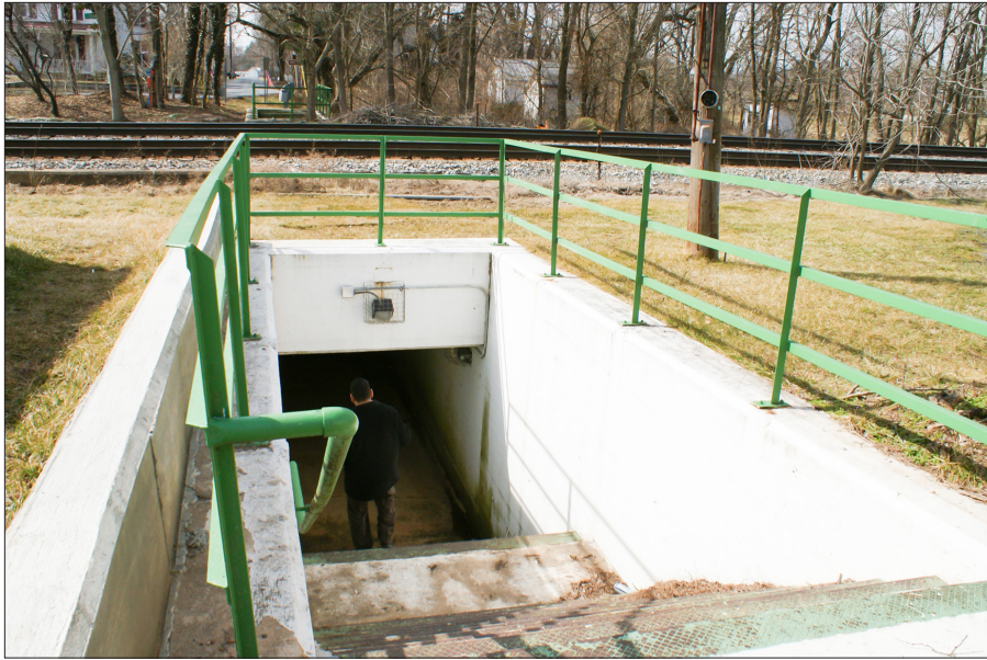
Pedestrian underpass connects both sides of the tracks at Boyds MARC Station
