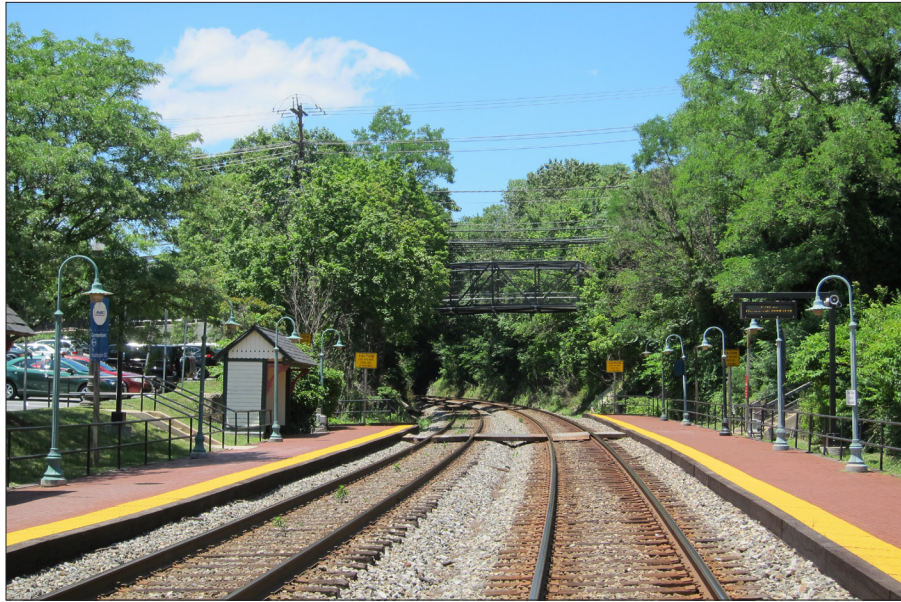
Germantown MARC Station and pedestrian bridge
