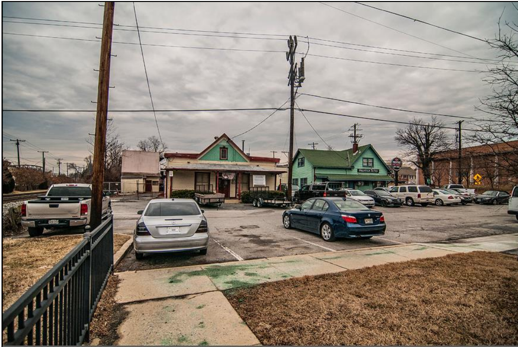
Figure 3: St. Paul Street with the two existing historic buildings to be retained (looking west)
