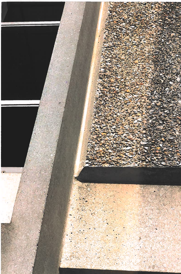
28. 900 Spring Street, Silver Spring, MD – John H. Sullivan, Jr., 1964 Detail of smooth and exposed aggregate concrete Photograph by Anne H. Adams, August, 2019
