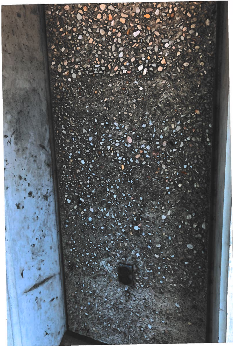
15. 900 Sprig Street, Silver Spring, MD – John H. Sullivan, Jr., 1964 detail of exposed aggregate concrete on first floor Photograph by Anne H. Adams, August, 2019
