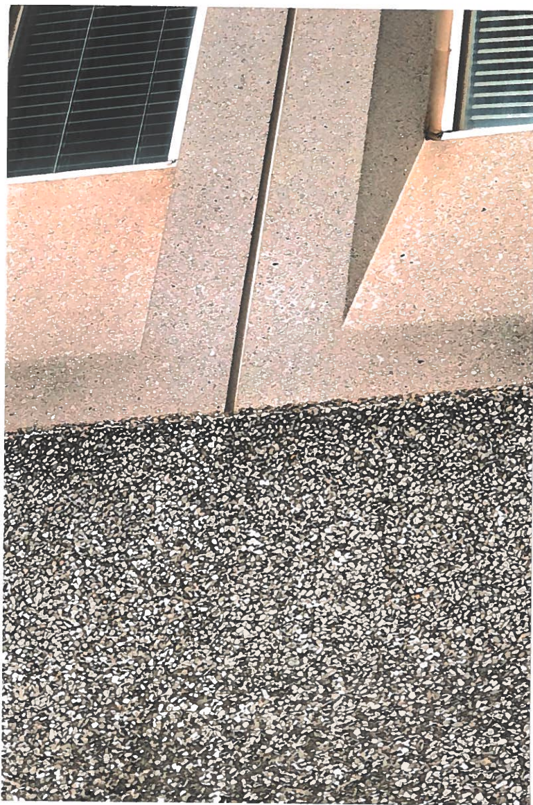
27. 831 East University Boulevard, Takoma Park, MD 1965 Detail of smooth and exposed aggregate concrete Photograph by Anne H. Adams, September 2019
