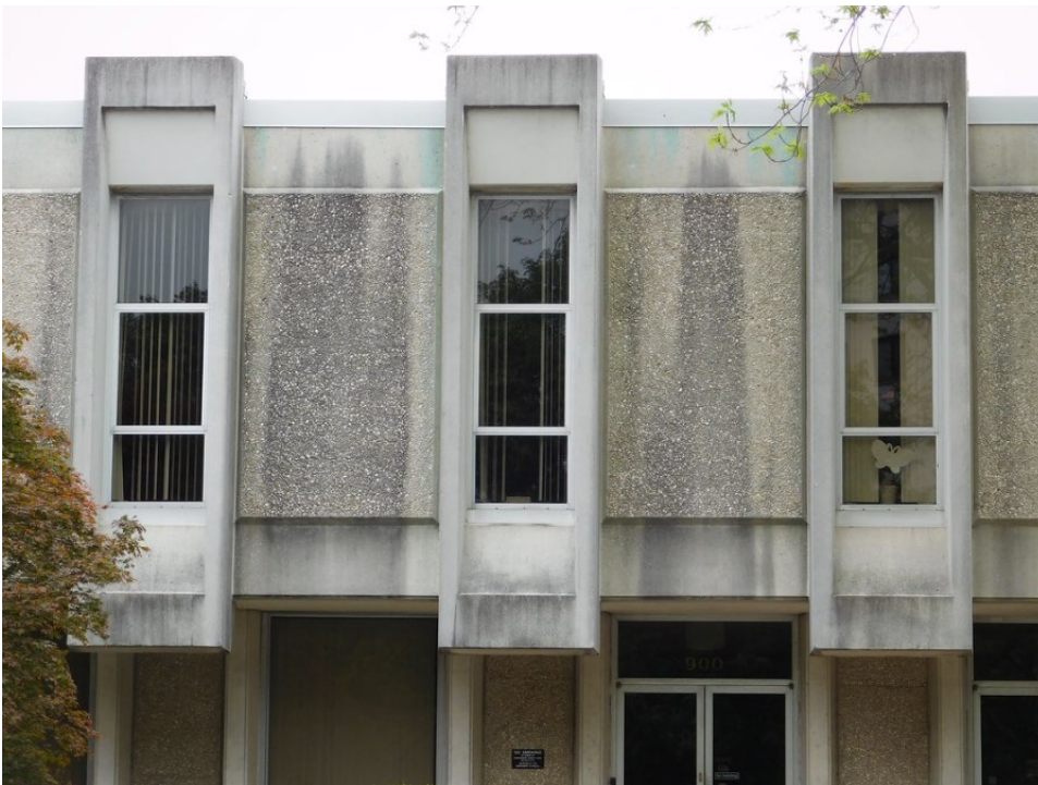
Figure 6: Detailed view of the second-story windows and exposed aggregate panels.
