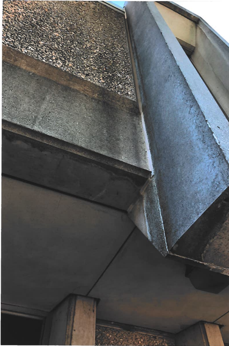
17. 900 Spring Street, Silver Spring, MD – John H. Sullivan, Jr., 1964 Detail of façade showing smooth and exposed aggregate concrete Photograph, Anne H. Adams, August, 2019
