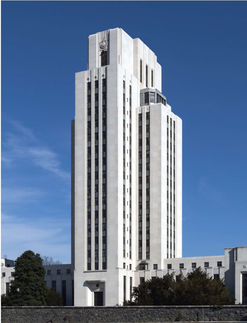
FIGURE 13: Naval Hospital Tower Building, 1942. Precast exposed aggregate concrete panels designed by John J. Earley. Paul Philippe Cret, architect. Carol Highsmith, photographer, 2014.
