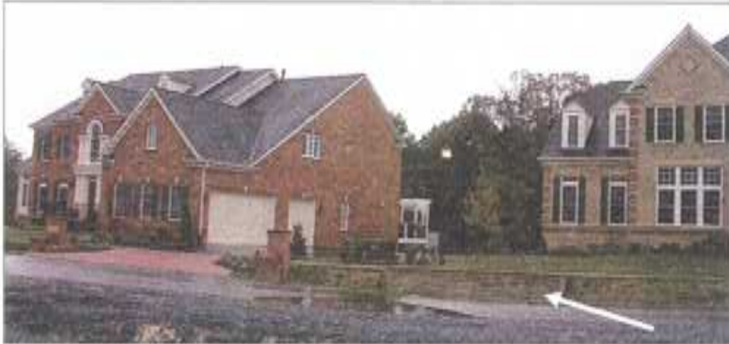
Figure 2 - Brick retaining wall on Lot 13
