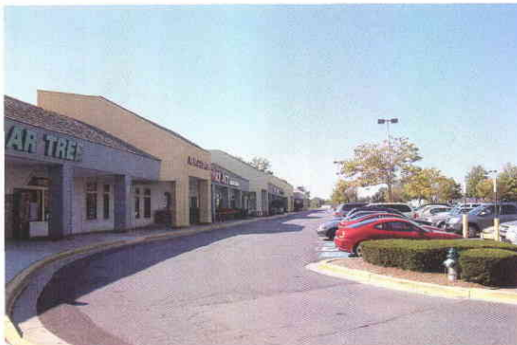
View of existing storefronts on the southeast.
