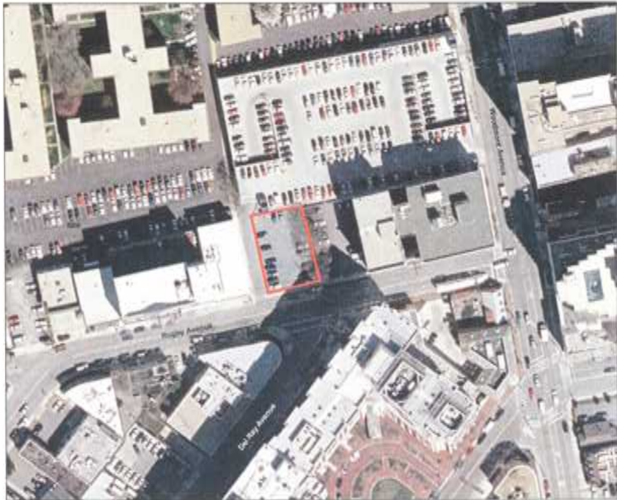
Site Aerial View
