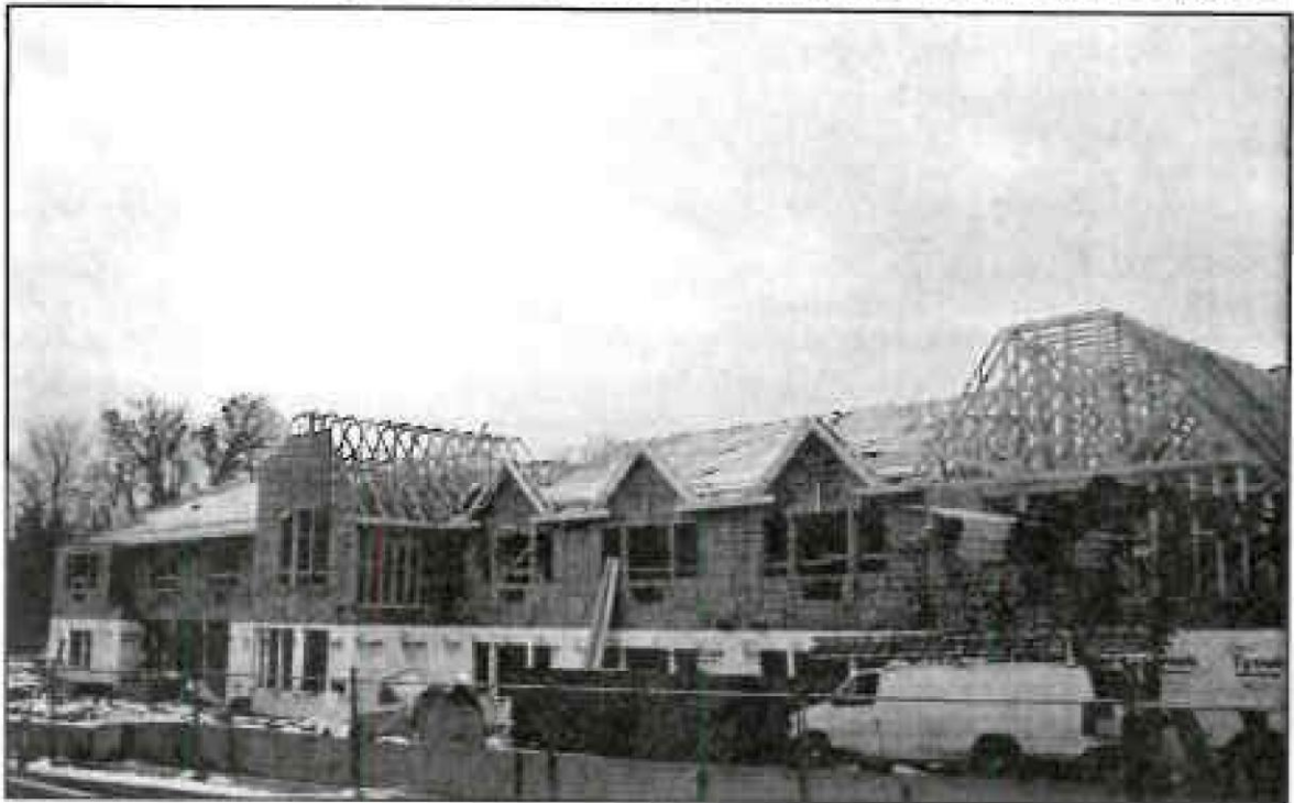
Grace House Assisted Living Facility in Silver Spring, Maryland.
