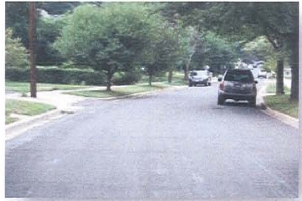
Figure 1d: Southwick St, looking west (towards Grant St)
