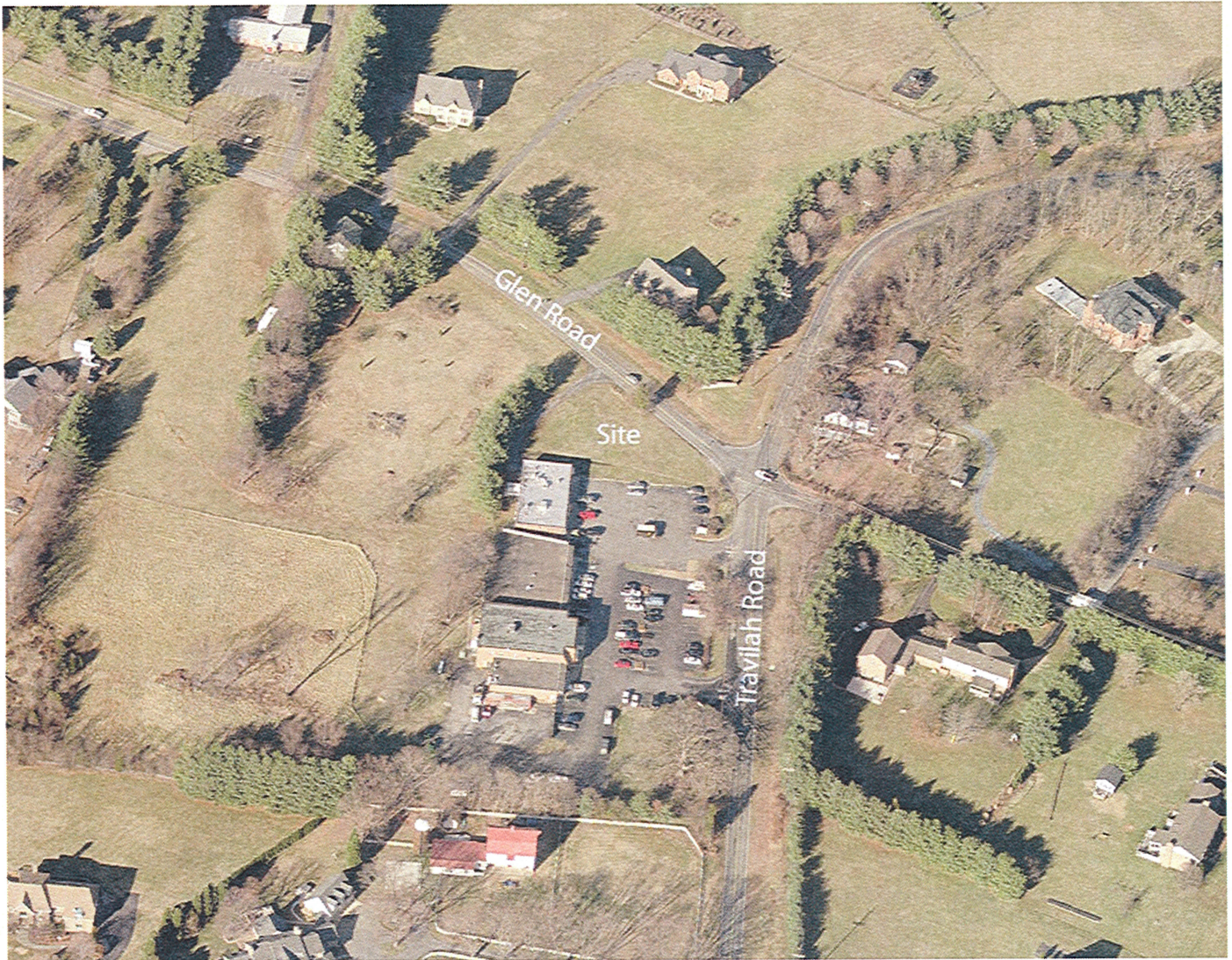
Aerial Site View
