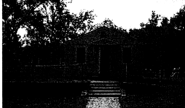
Figure C-1: Ken-Gar Palisades Recreation Building
