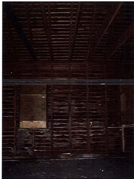
Picture #2: Stud wall, ceiling joists and roof rafters of the historic garage-Maintenance/Vehicle storage. Deteriorations in siding is visible from inside
