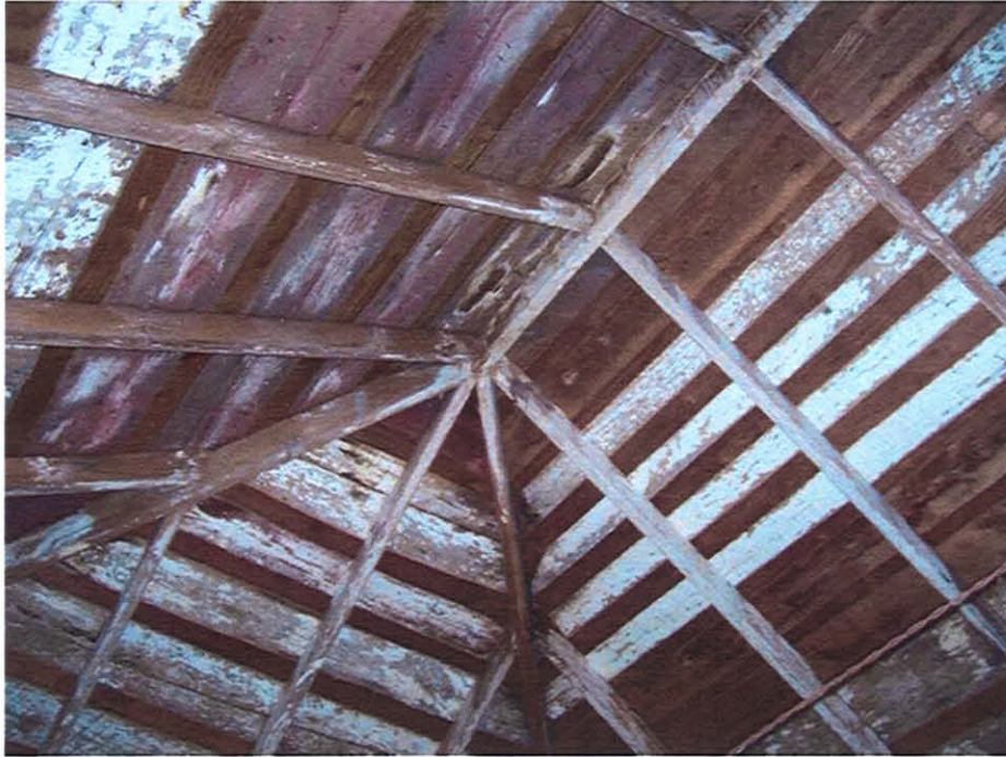
Picture #13: Roof construction system of the historic farm outbuilding
