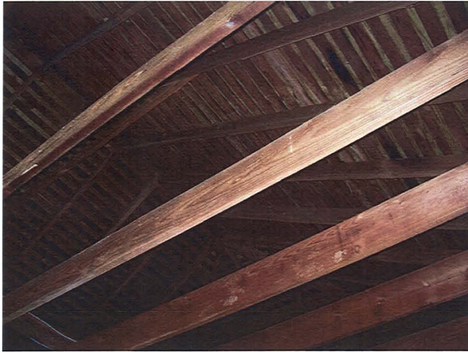
Picture #1: Roof construction system of the historic garage-Maintenance/Vehicle storage
