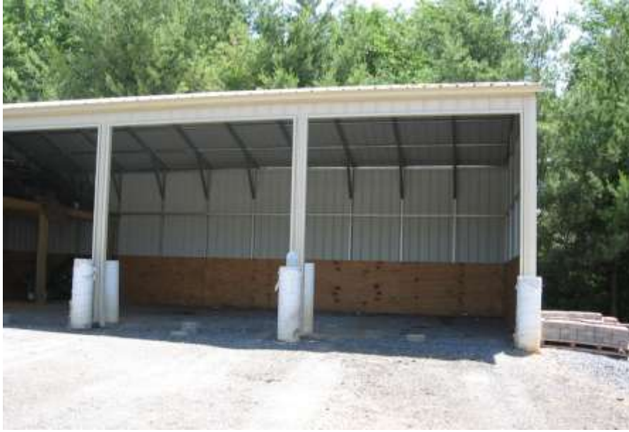
A building used to store equipment. This building will be removed.
