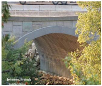
An example of a bottomless culvert, which is recommended for parcels 131 and 133
