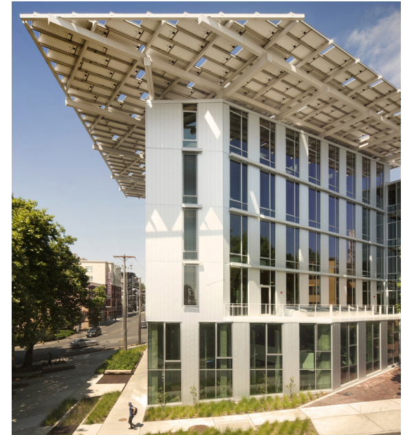
The Bullitt Center in Seattle produces all its energy on site using a rooftop solar array
