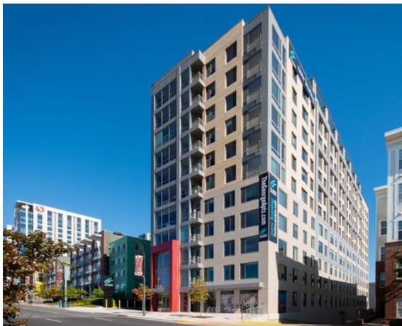
The George in Wheaton reused an existing office structure and converted it into a residential building by adding more floors on top
