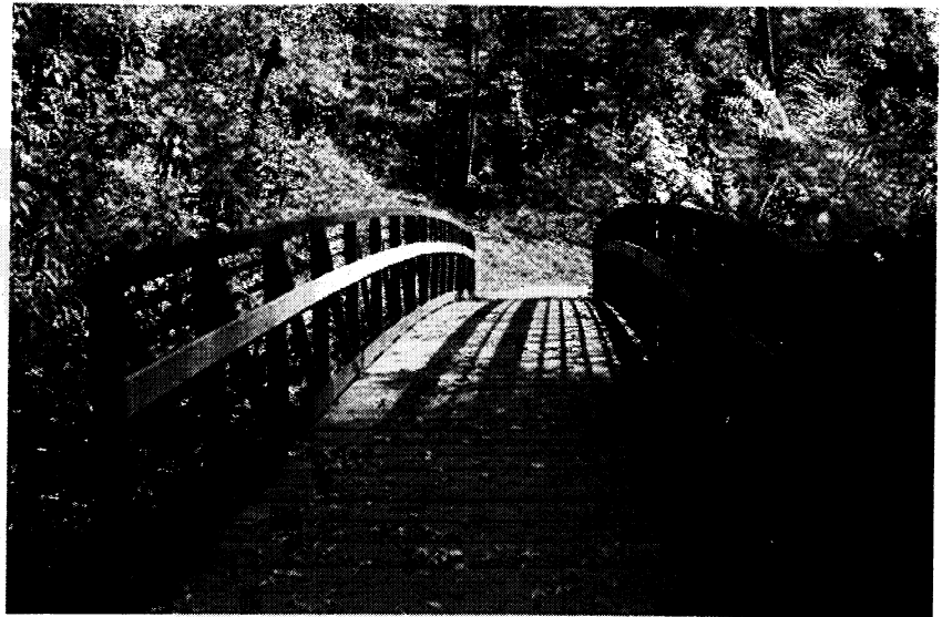
Figure 6 - Existing Bridge just west of Aspen. The bridge is 10' wide.
