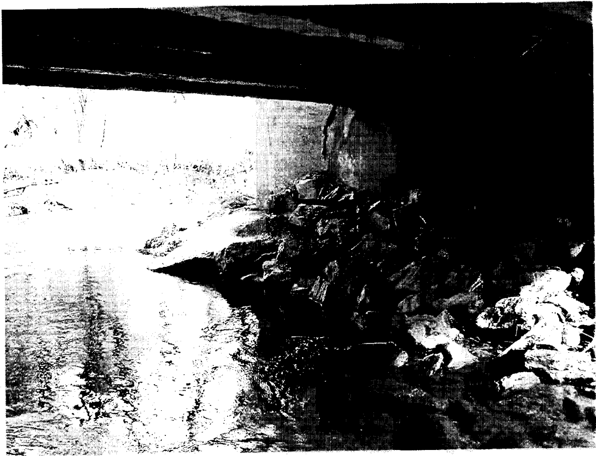
View of stream scouring the bridge
