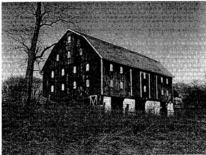
Barn, southeast corner
