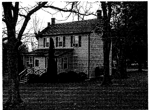
Rear façade, as seen from Dunnivant Drive approach
