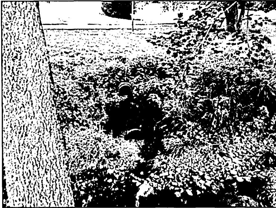
Figure 25 – Mutual 8 outfall pipe broken off and scour in stream.
