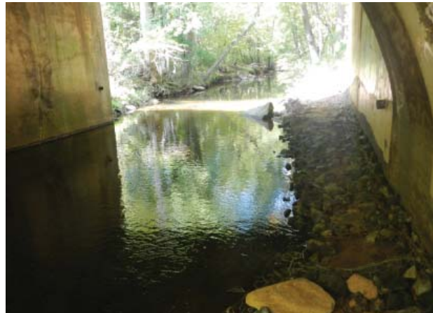
Gabion baskets line one side of the North Branch as it goes under Muncaster Mill Road.
