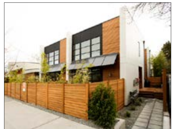
Solar panels awnings on these townhouses provide electricity and shading from western, summer sun.
