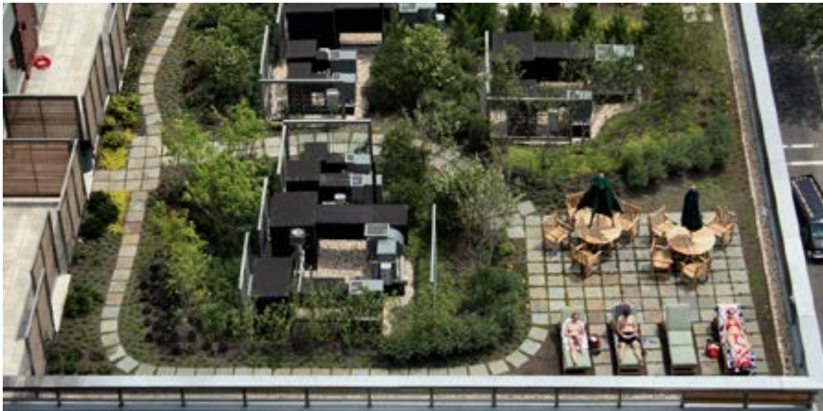
Vegetated roofs can be much more than sedum planted in a 4 to 8 inch medium. This roof includes pervious pavers, perennial plants, shrubs and small trees in deeper soil medium.
