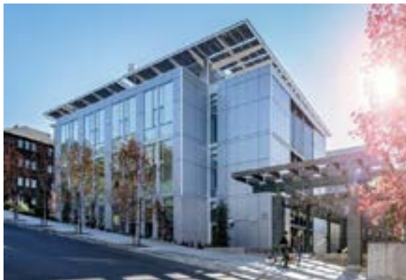
Solar panels incorporated into the design of this office building provide energy generation on site.
