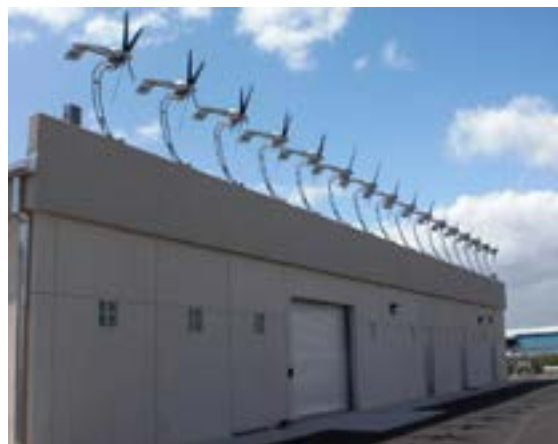
Micro-wind turbines on buildings are becoming more efficient and cost competitive.
