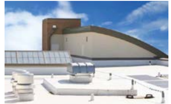
Cool roofs reflect up to 90 percent of the sun's energy, reducing energy consumption to cool the building.
