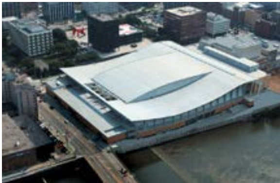
This curvilinear roof was created with a cool roof system to help minimize heat island effects.
