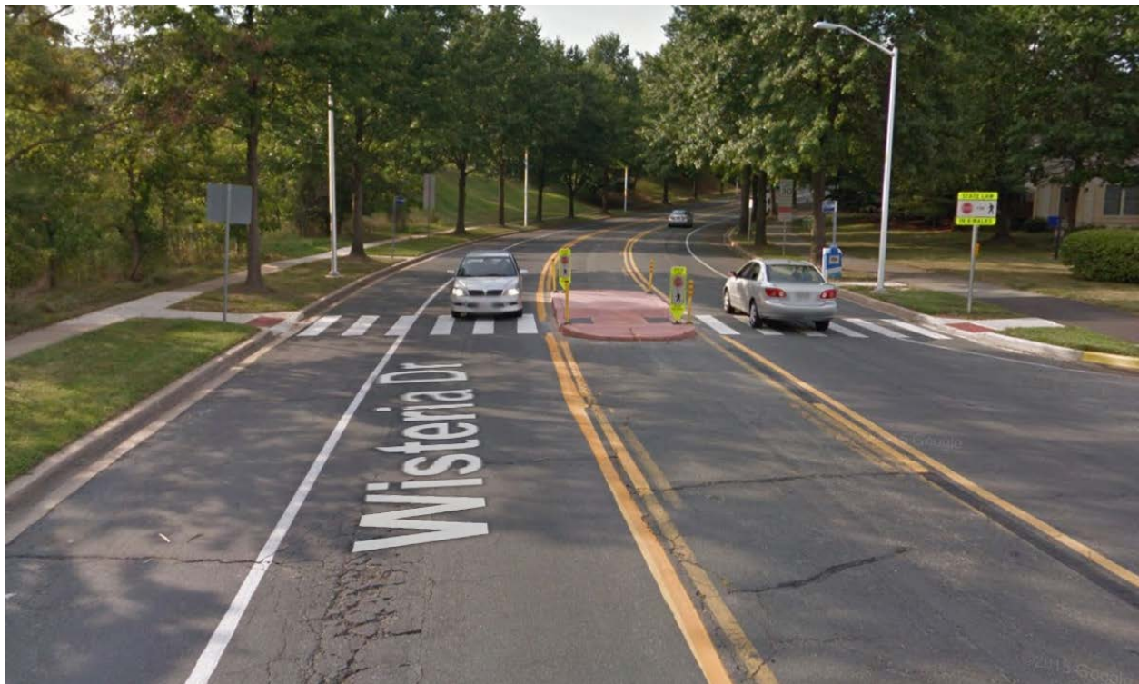
A pedestrian median refuge on Wisteria Drive south of Christa McAuliffe Elementary School
