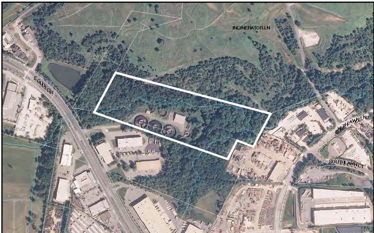
Figure 2 Existing Abandoned WWTP at Gude Drive
