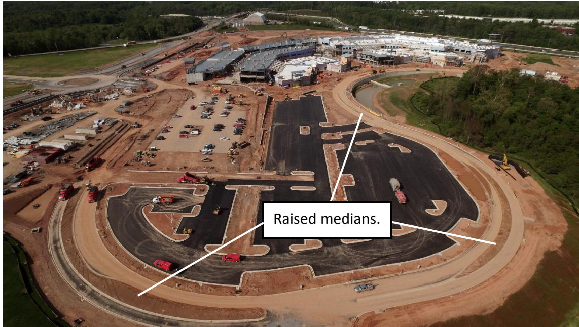
Figure 5. Mall site during construction showing the constructed raised medians. The construction truck on the left appears to fill the entire lane.
