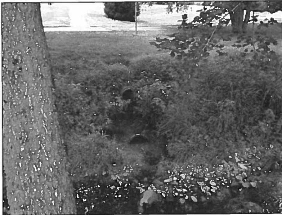
Figure 25 – Mutual 8 outfall pipe broken off and scour in stream.
