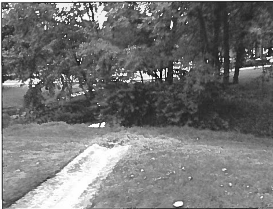
Figure 18 – Mutual 8 concrete conveyance of runoff from parking lot.
