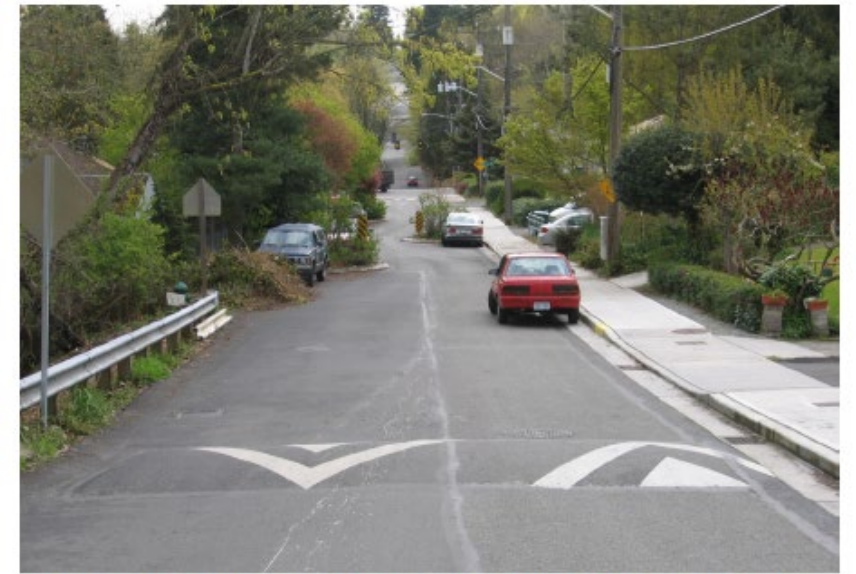
Speed Hump showing drainage bypass along curblines and chine in background (Seattle, WA)
