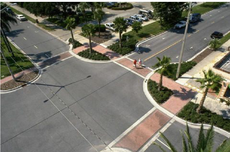
Figure 3.21: Bulb-outs create shorter crosswalk distance for pedestrians
