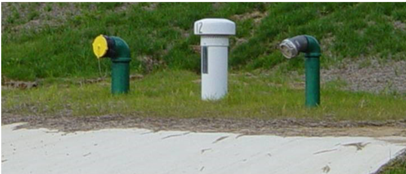
Figure 3.29: Hydrants connect to underground water tanks and provide access for fire department personnel
