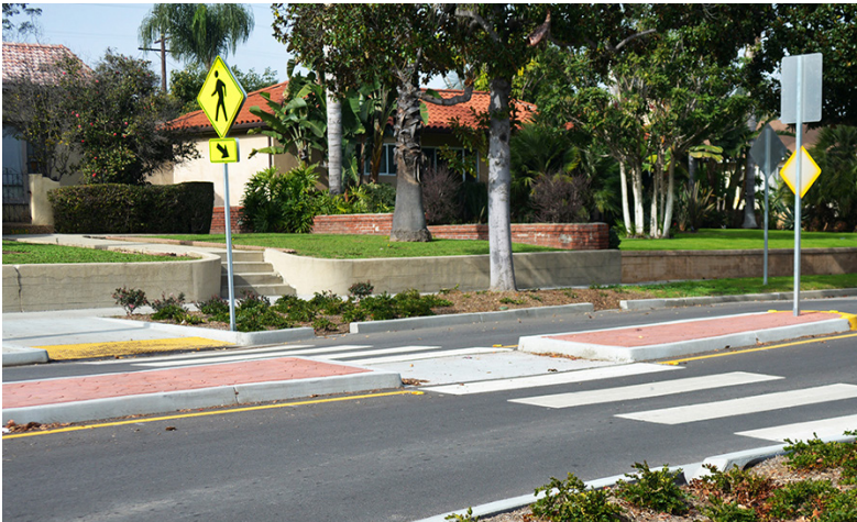
Figure 3.25: Median refuge islands reduce pedestrian exposure when crossing roadways and can be designed with mountable curbs to support Fire Department access
