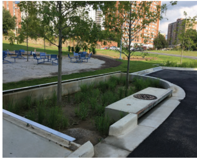
SECTION: STORMWATER INFILTRATION PLANTER
