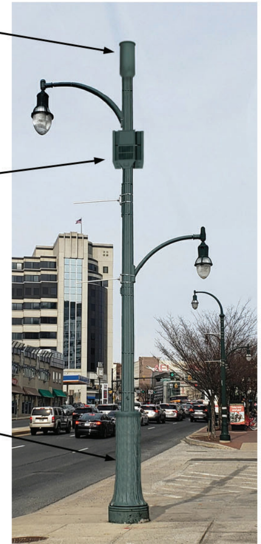
4G & 5G Antennas Mounted on Teardrop Luminaire Pole Above and Below Light with Equipment Base
