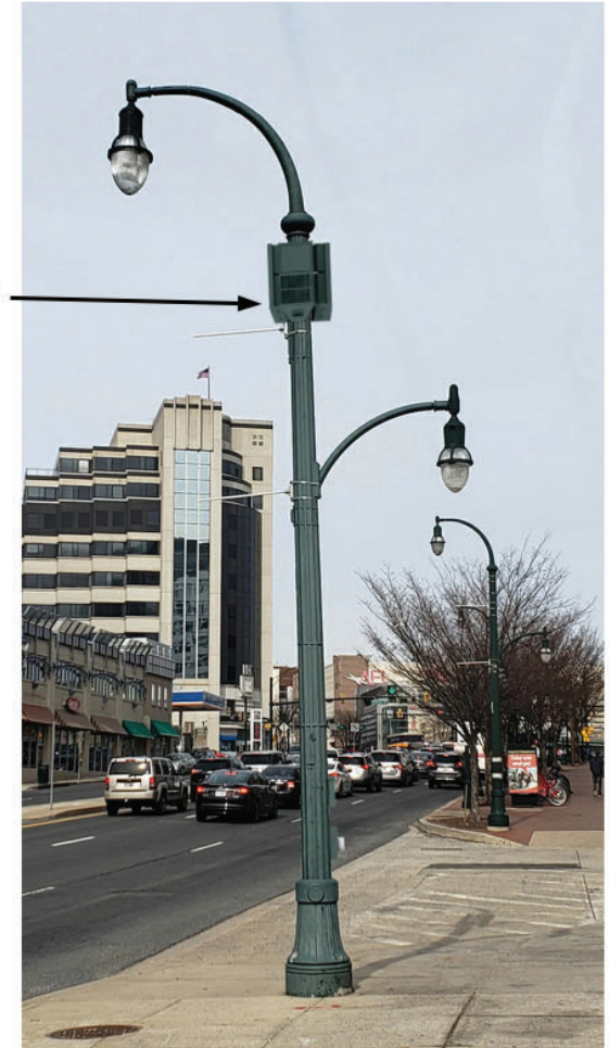
5G Antennas Mounted on Teardrop Luminaire Pole Below Light
