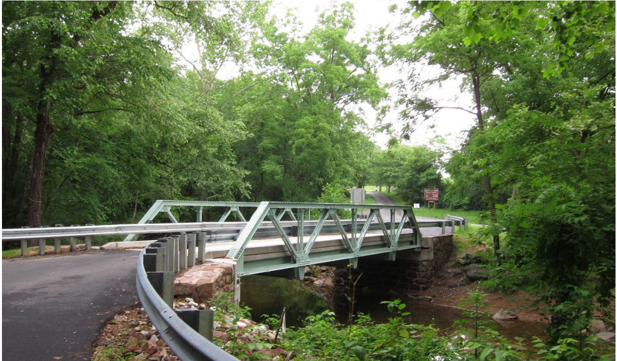
Preservation of this 1910 pony truss bridge which crosses the Dry Seneca Creek on Exceptional Rustic Montevideo Road was a factor in creating the program.
