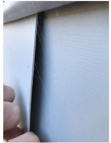
Beaded vinyl siding on front of Lot3; NOTE: Typical for all 3 Lots where "hardy/ cement plank siding is required per Resolution.
