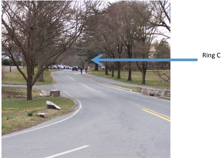
Figure 5 View from East-West Highway & Meadowbrook Lane looking south towards Ring C proposed site Feb 16 2020
