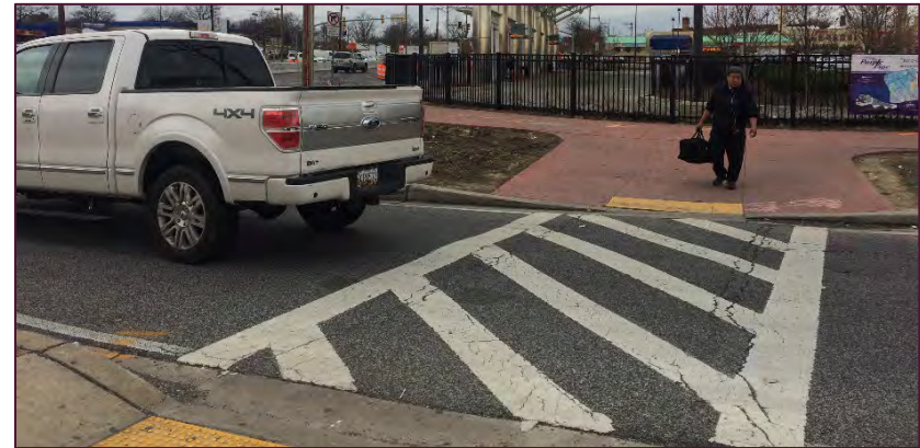
Figure 22. A channelized right turn immediately adjacent to the busy Takoma-Langley Crossroads Transit Center.
