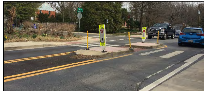
Figures 14 and 15. The crossing at Bonifant Street and Dale Drive, top, would benefit from the traffic-calming treatment at Mansfield Road and Dale Drive, bottom, applied to most four-way intersections of Dale Drive south of Wayne Avenue.
