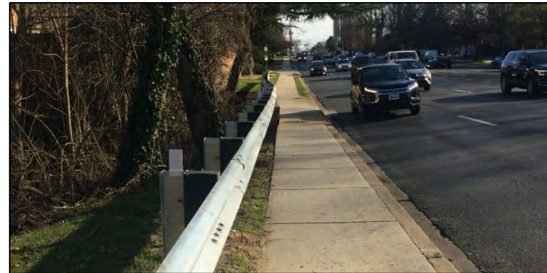
Figure 4. The Connecticut Avenue sidewalk at Chevy Chase Lake Drive, by the future station entrance, has no buffer between pedestrians and a major highway with a 35-mph posted speed limit.
