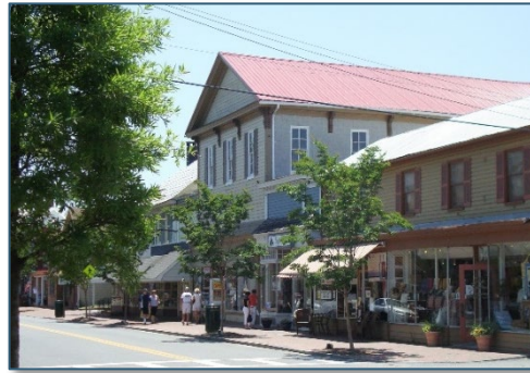
Buildings have varied and simple roof lines along streetscape
