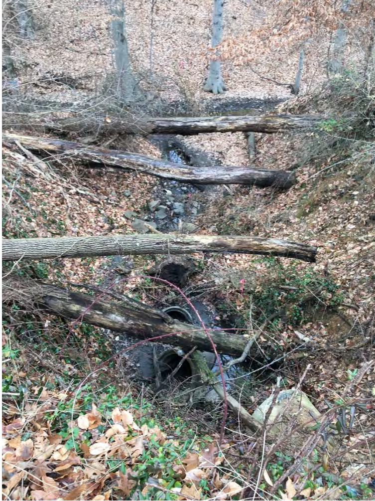
Figure 20: Degraded Outfall Flowing Into Larch Tributary
