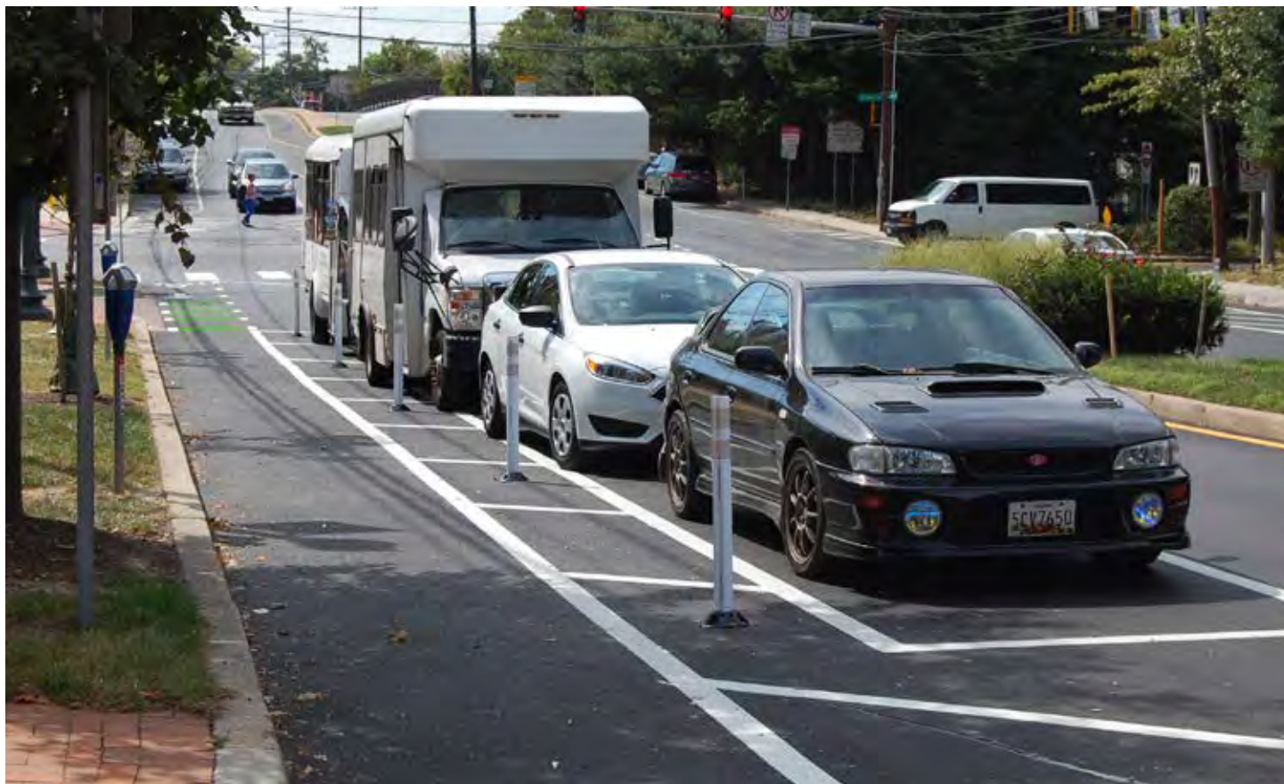
Parked cars provide separation from traffic for this bike lane in Silver Spring, MD.
