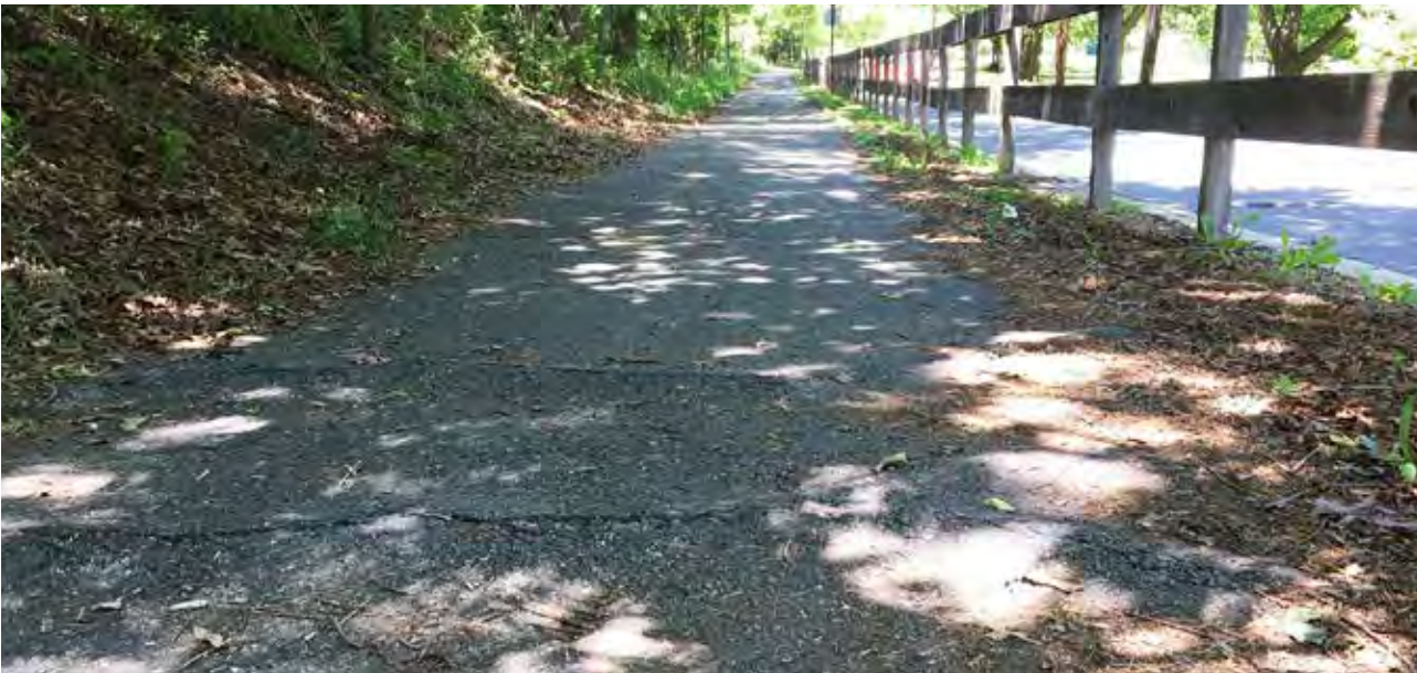
Pavement cracking is common on sidepaths
