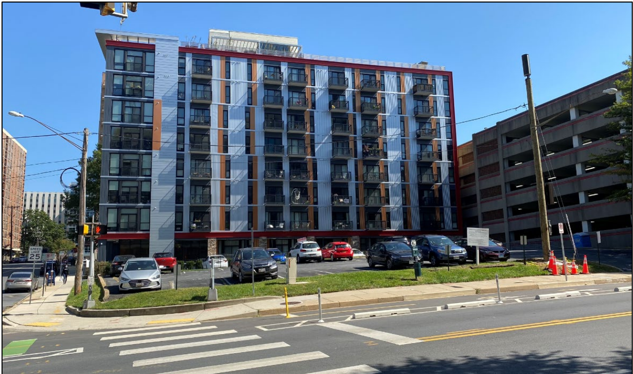
Figure 5: Second Avenue Frontage (Looking east)
