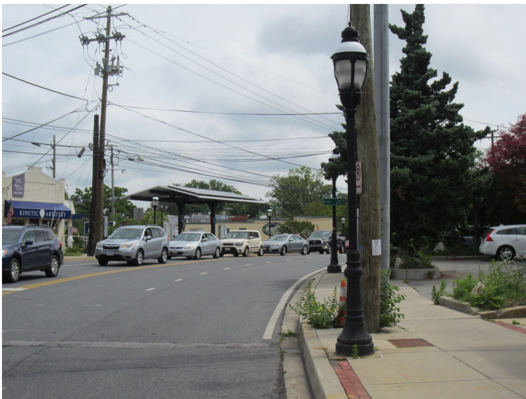
Picture 4 – Stopping Sight Distance Limited by Utilities and Vegetation
