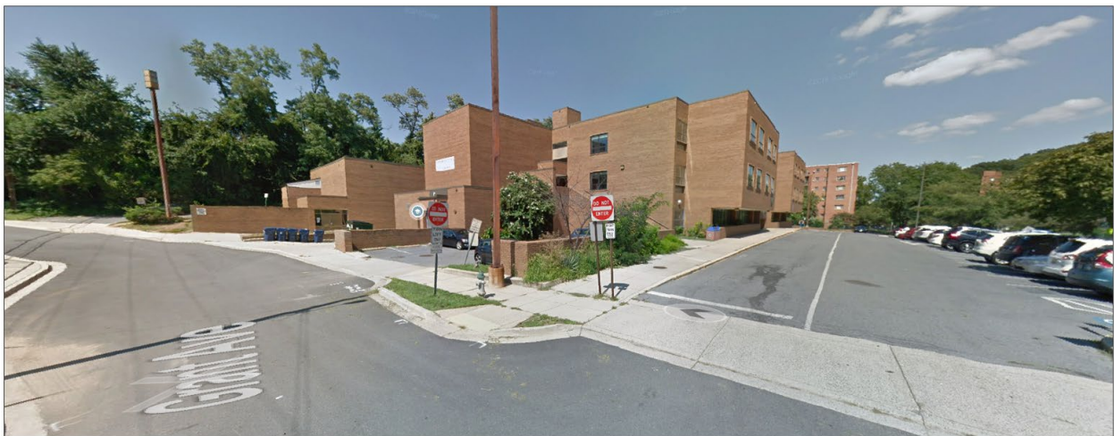
Figure 5: North facing view of Piney Branch Elementary School on opposite side of Grant Ave
