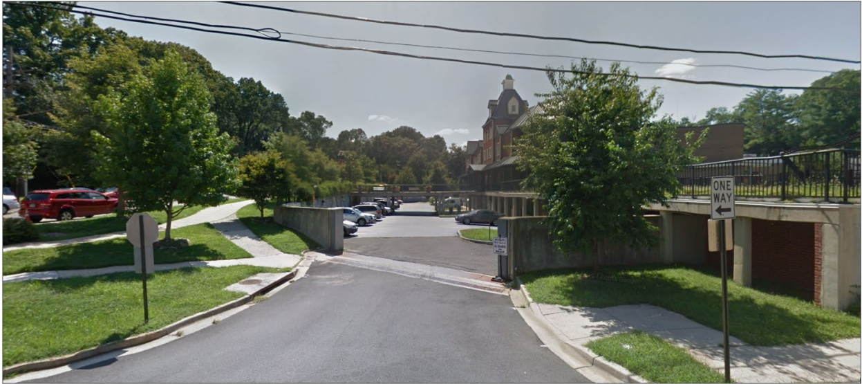
Figure 4: Southeast facing view of lower parking lot (floodwalls and open floodgate in center of image)
