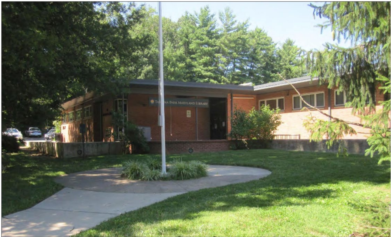
Figure 2: Existing Library Building to be Demolished
