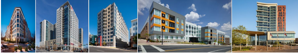
Wheaton recent development, from left: Solaire Wheaton, The Exchange, The George, AVA Wheaton, M-NCPPC HQ
