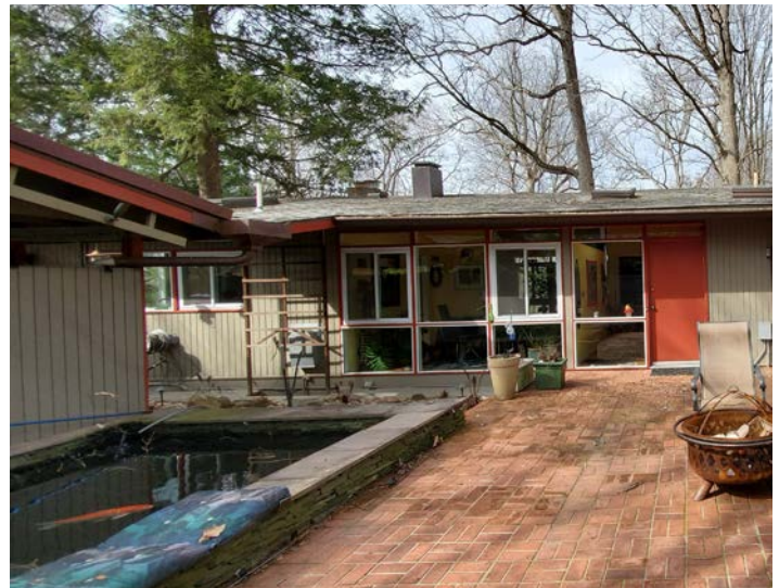
Figure 44: Example of brick paver patio.
