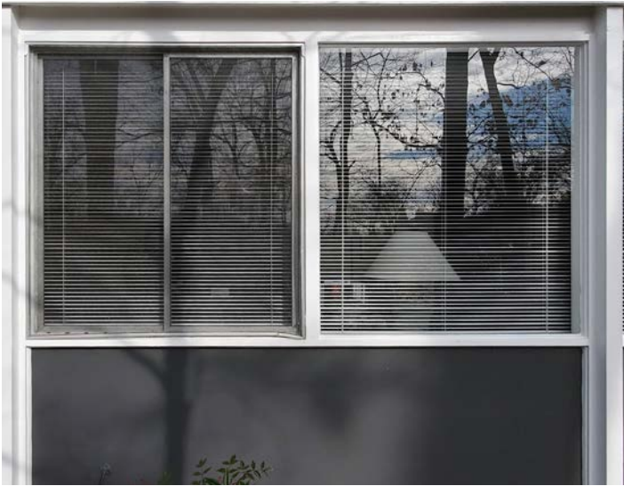
Figure 16: Example of a typical window (left) and non-compatible replacement window (right). Note the differences in the design, dimensions, and material of the trim.
