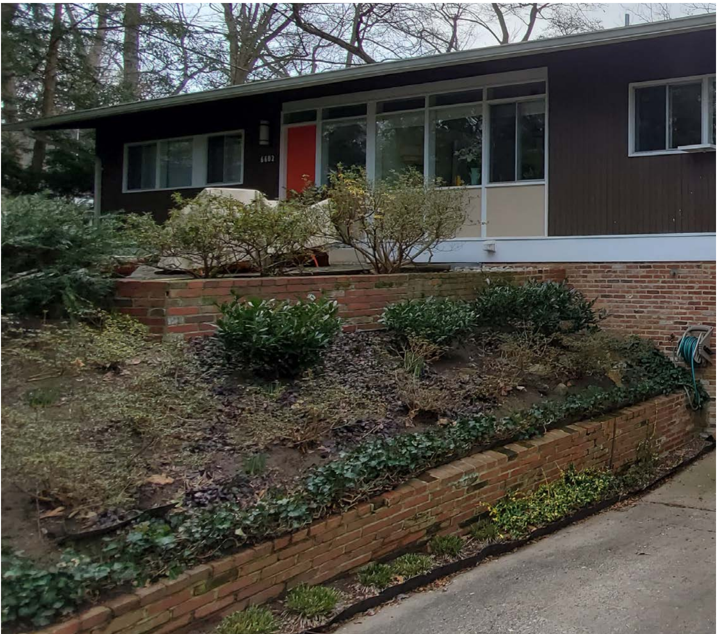
Figure 46: Example of brick retaining walls.
