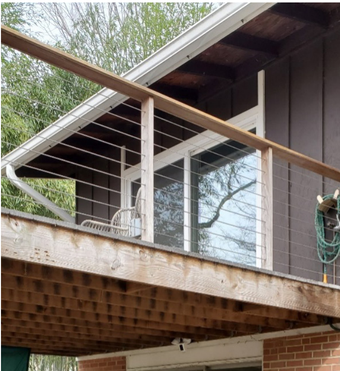
Figure 29: Example of a compatible deck-mounted railing system at 6604 Virginia View Court.
