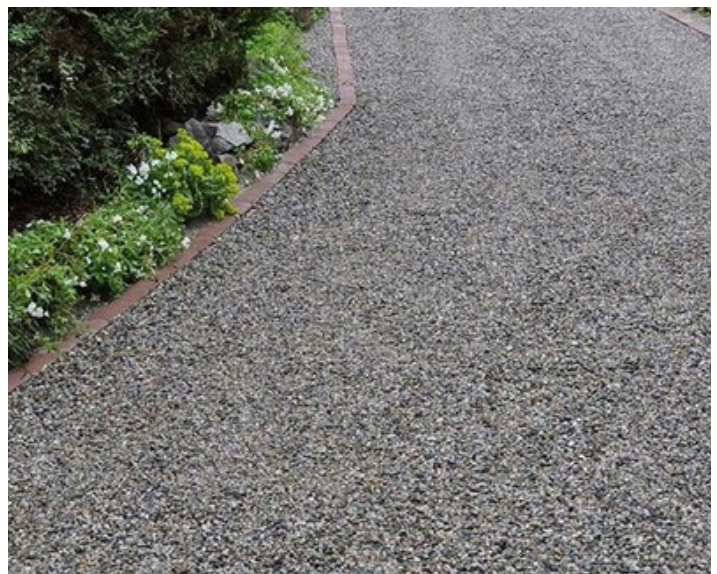
Figure 40: Example of a 3/8" crushed stone driveway.
