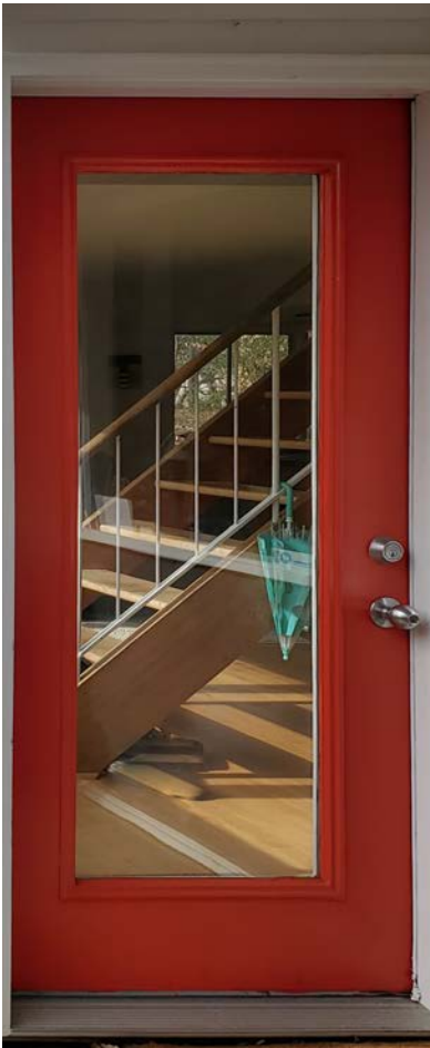
Figure 12: Example of single-light entrance door.
