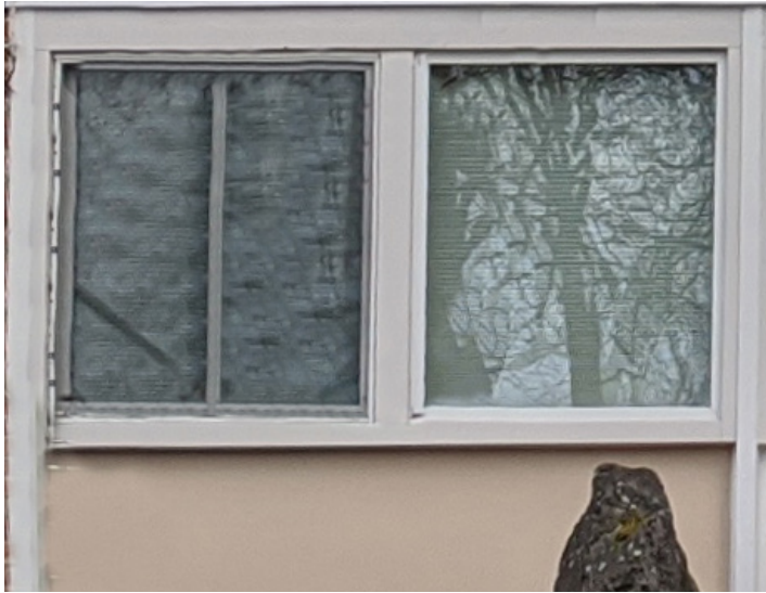
Figure 16: Example of a typical window (left) and non-compatible replacement window (right). Note the differences in the design, dimensions, and material of the trim.
