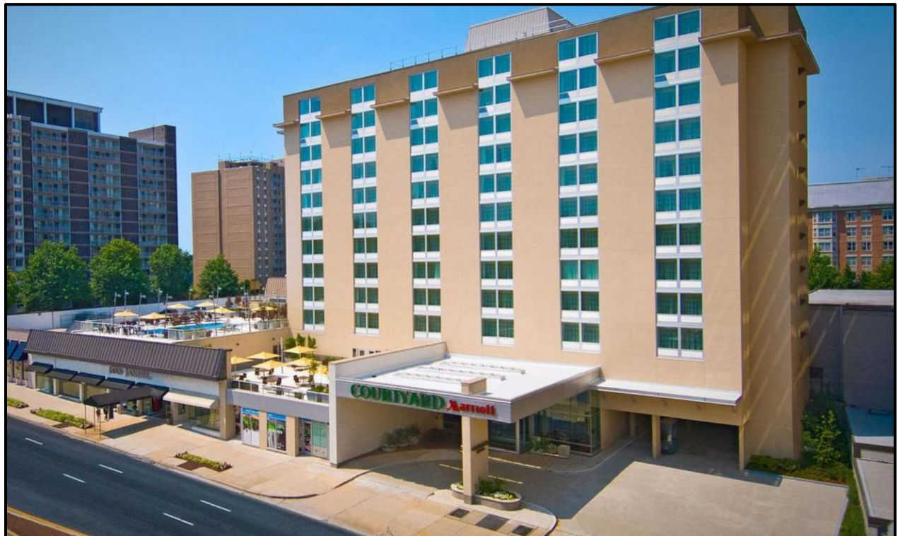
Figure 3 – Existing building viewed from Wisconsin Avenue, with the 12-story hotel and adjoining 1-story retail with structured parking
