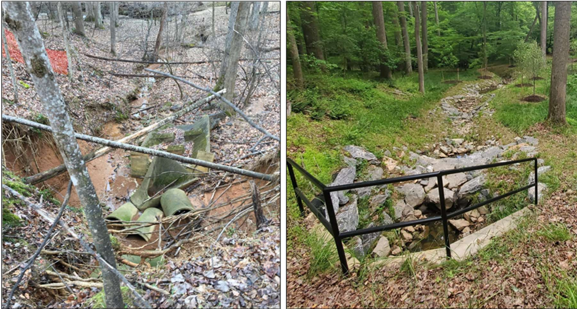
Before and after photographs of a storm drain outfall channel restoration completed 2021 in Watts Branch SVU 3. Photos by Jacqueline Hoban.
