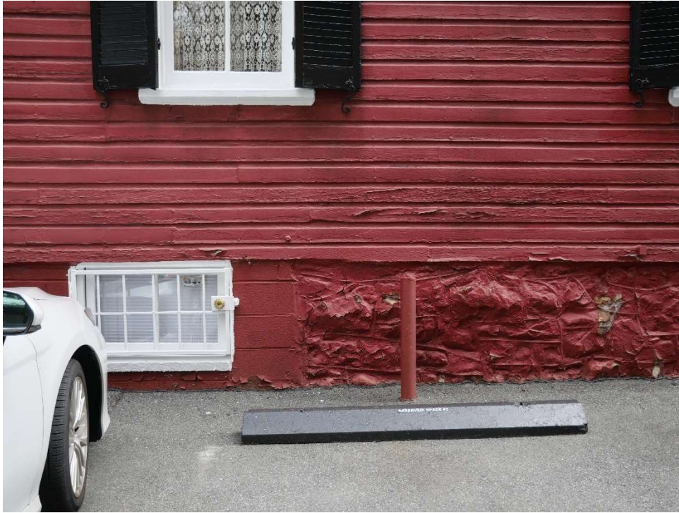
Figure 9: Detail of mixed foundation materials visible on the west-facing elevation.
