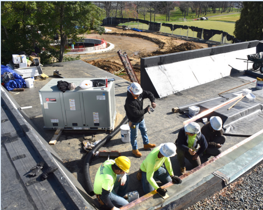
Construction workers affix copper flashing to a section of roof over the Maryland Room extension of Clubhouse I on April 11. The background, to the north, shows partial construction of a circular driveway situated between Clubhouse I and the space planned for a new Administration Building. Photo by Leisure World News
