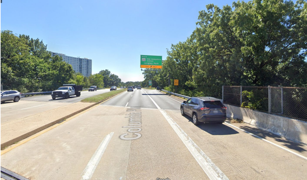
Image shows that southbound US 29 is currently reduced from three to two through lanes within the interchange with New Hampshire Avenue (MD 650).
