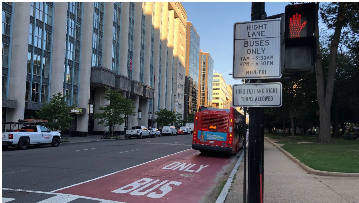
Curb Lane Transitway in Washington, DC
