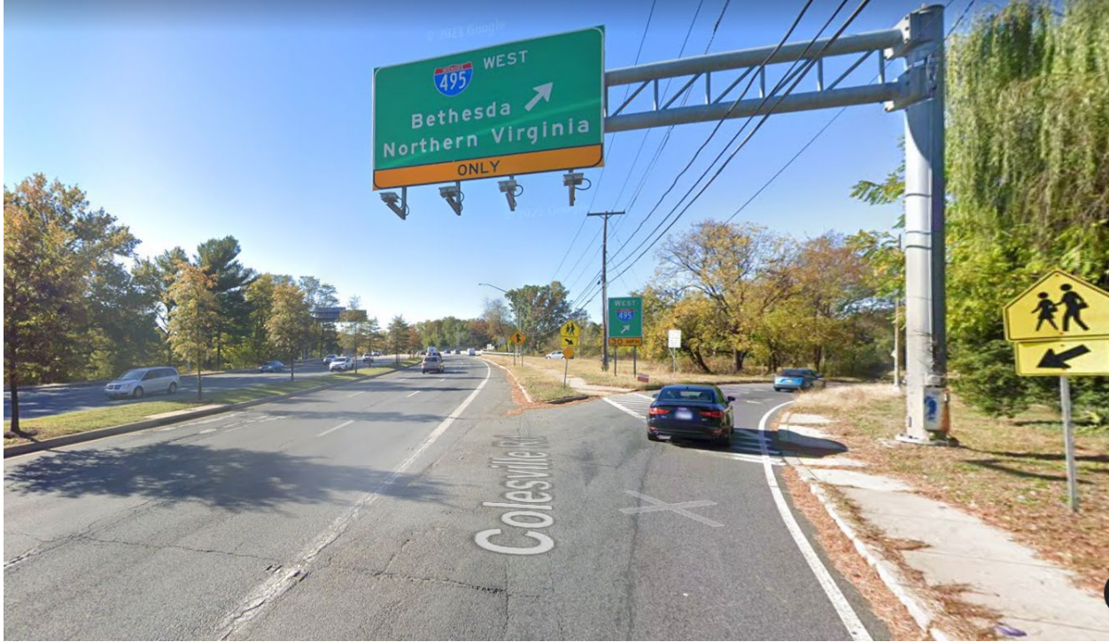
Image shows southbound US 29 at the I-495 ramp. The ramp is proposed to be widened from one to two lanes.
