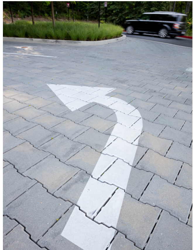
The parking lot at the Brookside Gardens Visitor Center uses permeable interlocking pavers for the parking spaces (Montgomery Parks).
