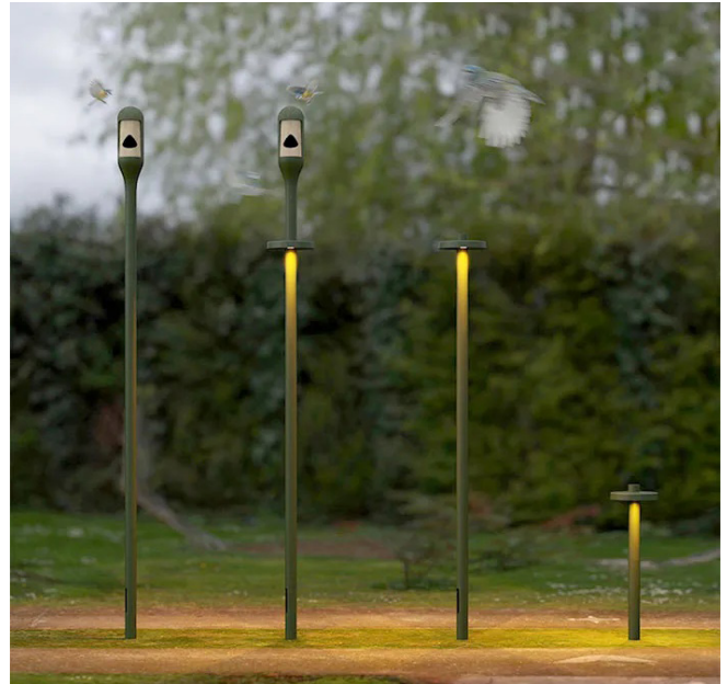
An example of bird-friendly lighting that illuminates the ground for safety and does not direct light upward (artemide.com).
