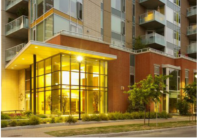
Transparency at public spaces on the ground floor . (Hobin Architecture)
