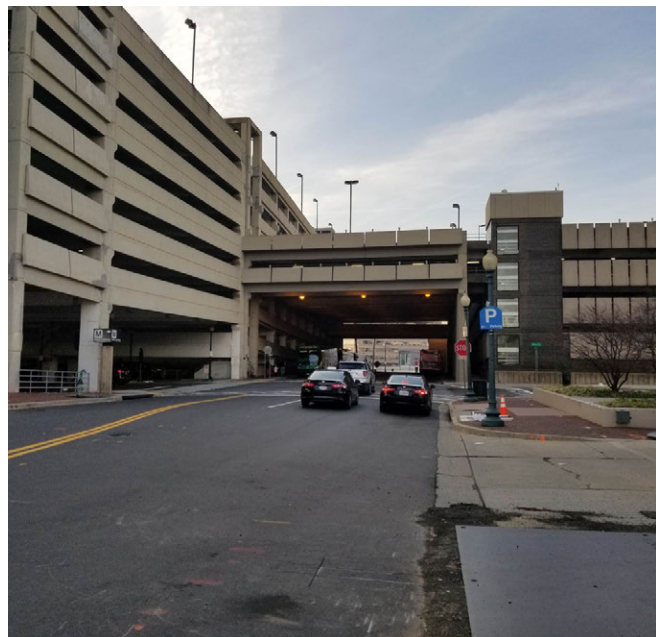
Existing conditions at Bonifant Street and the Bonifant-Dixon parking garage. View looking east down Bonifant Street (top), view looking west towards the Transit Center (bottom).
