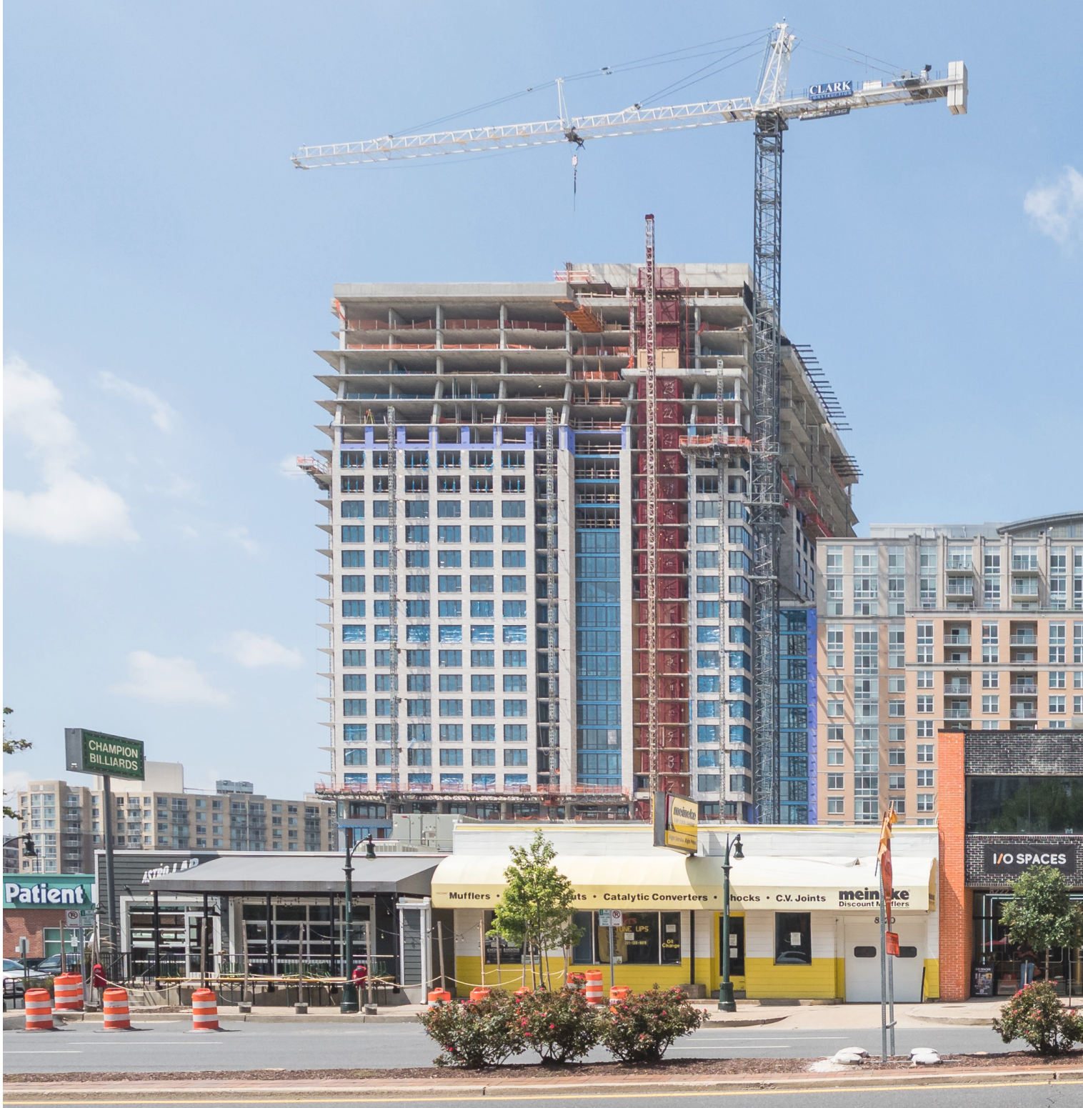
View of construction in the Ripley District, from Georgia Avenue.
