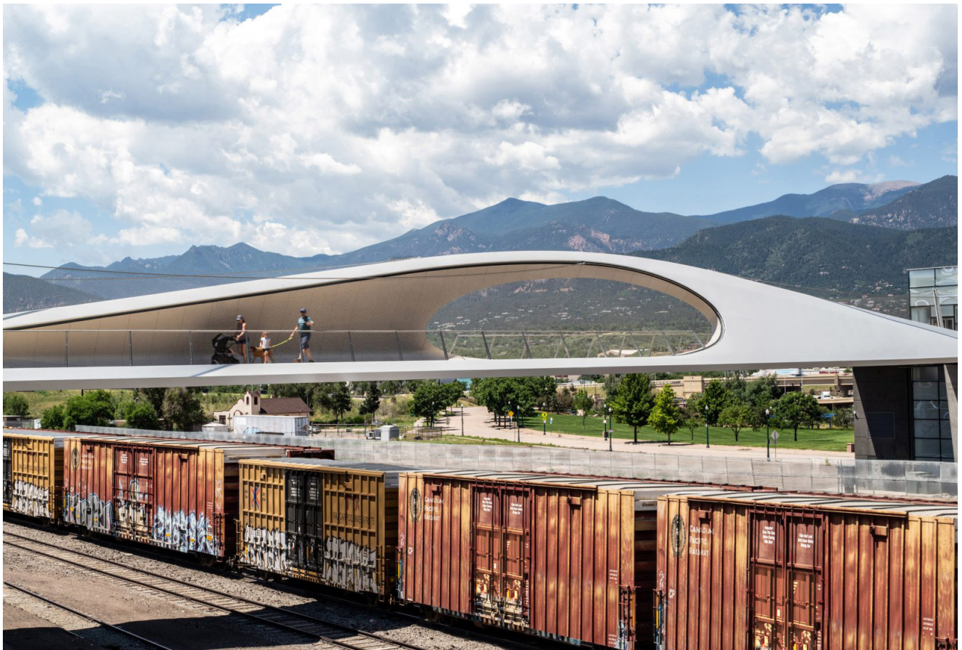
Bridge crossing over rail in Colorado Springs, CO completed in July 2021.
