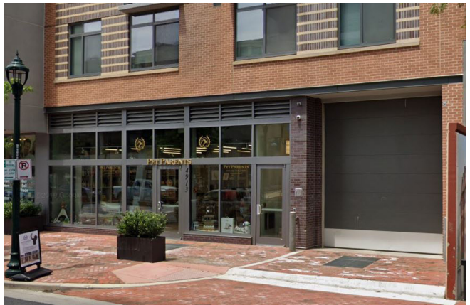
Service entrances in Bethesda. Note that the sidewalk materials are carried across the driveway entrance so the pedestrian experience is continuous.
