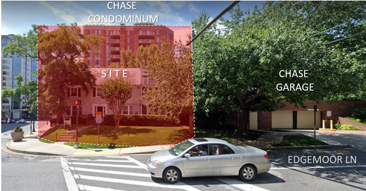
Figure 3: Edgemoor Lane Frontage (Looking South)
