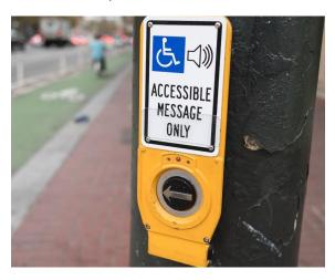
An accessible pedestrian signal reads "Accessible Message Only" and has a confirmation light. Photo Credit: SFMTA
