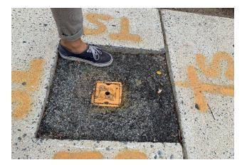
A poorly filled utility cut in the sidewalk. Shoe for scale.
