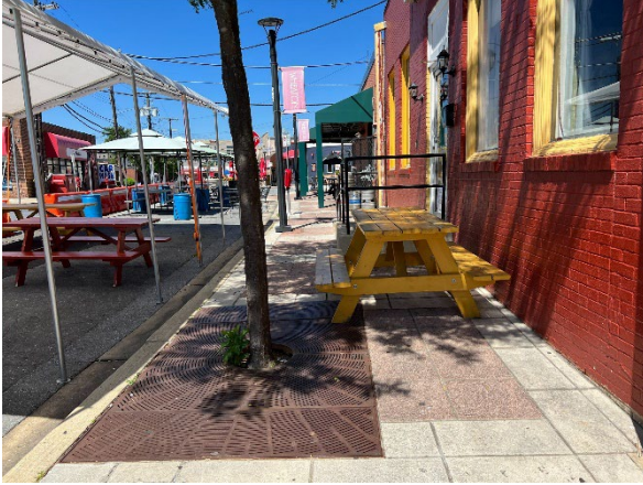
Pedestrian space is made inaccessible by a table and a tree.
