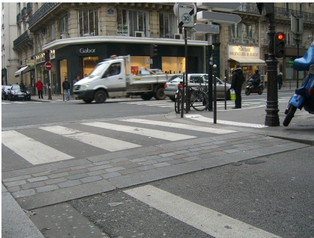
A raised crossing at sidewalk-level across a low-speed, low-volume street. Photo Credit: Vladimir Zlokazov
