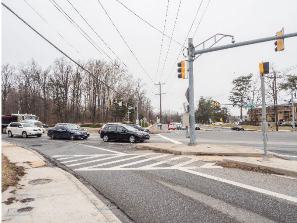
A channelized right turn lane with porkchop island at Bel Pre Road and Georgia Avenue
