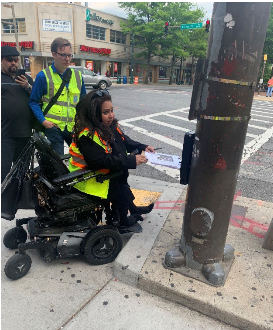
This pedestrian is unable to reach an APS in Downtown Silver Spring because the push button is located on a raised surface that her mobility device cannot navigate.
